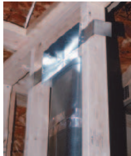
Figure 3. Each wall-mounted fresh-air and stale-air register requires a rectangular duct fitting called a stackhead. Stackheads are installed \frac{1}{2} inch proud of the joists, like electrical boxes.
